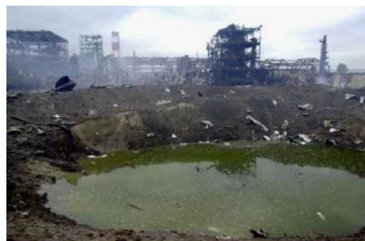
Fig. 1. Crater left by the explosion in Toulouse and damage.
